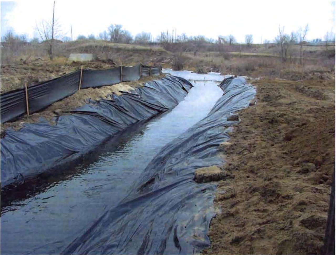
Lined Channel Diversion
