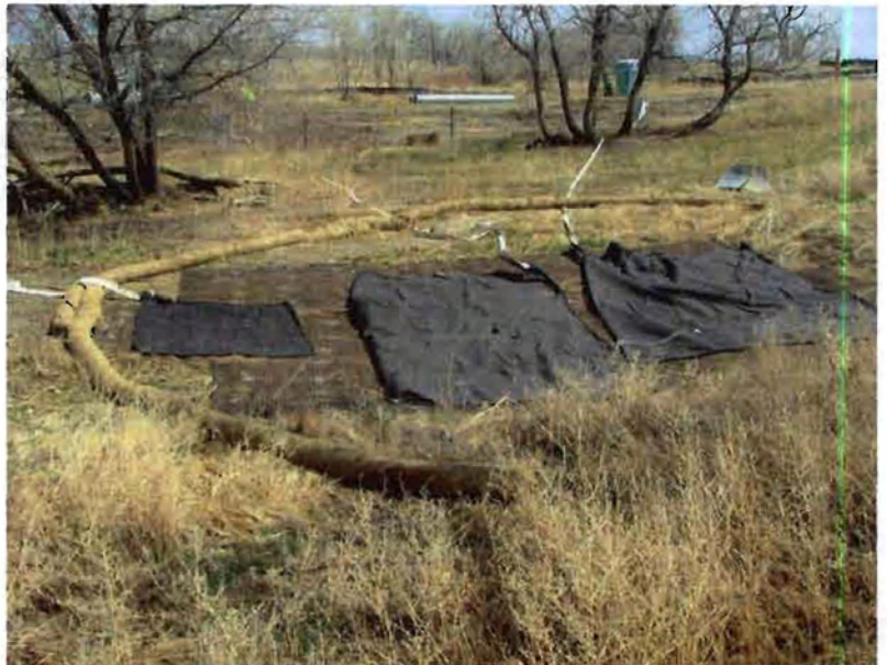
Discharge area established with filtration bags.
