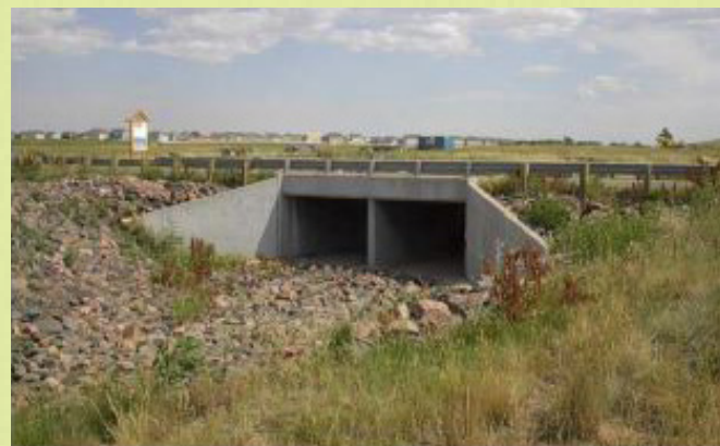
MISSISSIPPI AVENUE CONCRETE BOX CULVERT
