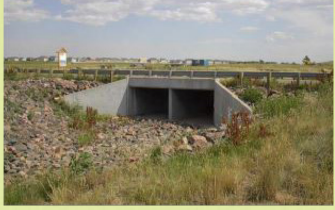
MISSISSIPPI AVENUE CONCRETE BOX CULVERT
