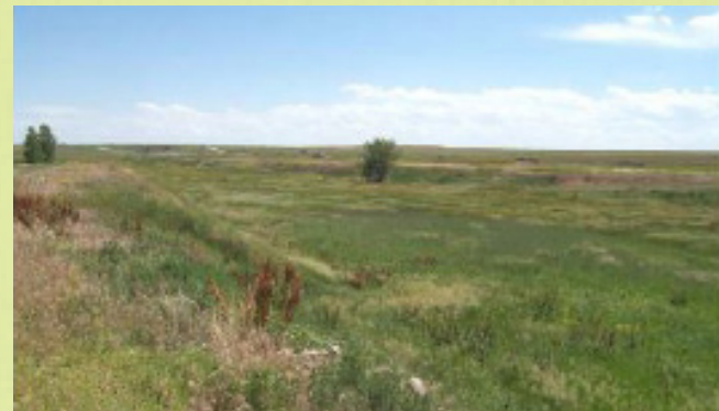
TRIBUTARY 3000W WITHIN THE CLOSED AURORA LANDFILL
