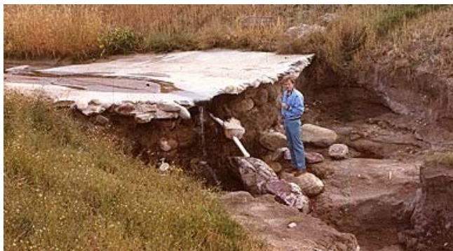
Figure 1. Typical stream degradation in Denver area after a watershed urbanizes.
