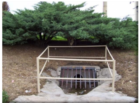
Outflow Structure (6CCC-OPB)
