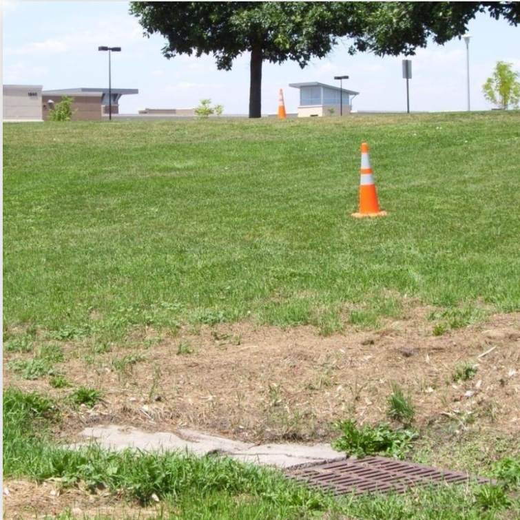
Below: One of the many low-flow grates inside and on the bottom of the pond
