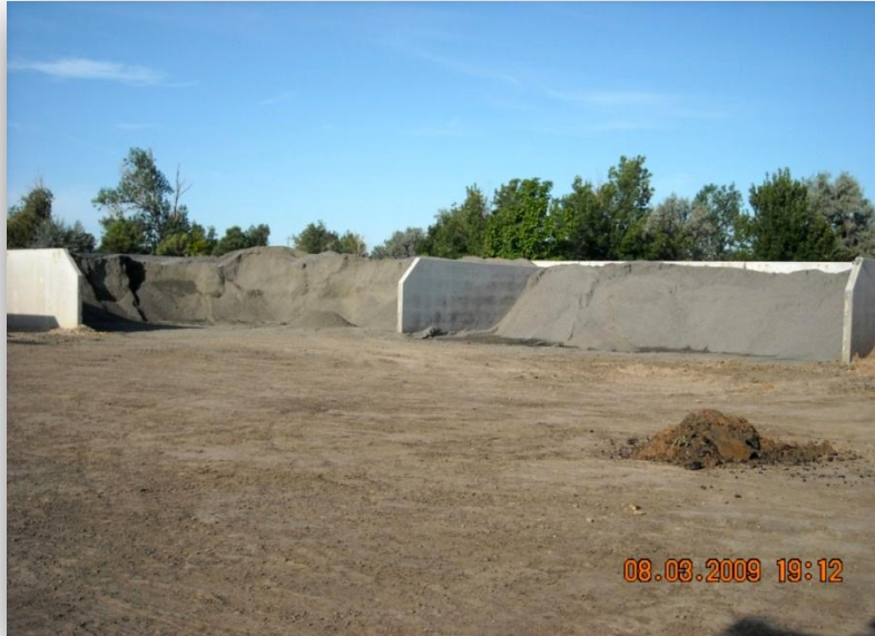
Water T & D's two main storages bins at the Southwest corner of Aurora's property.
