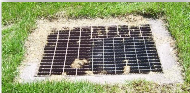
Below: One of the many low-flow grates inside and on the bottom of the pond
