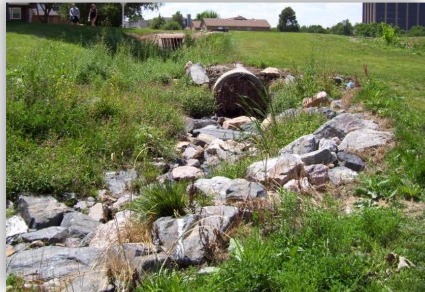
Below: Outfalls on the South side of the pond empty StormWater from the street into the pond,
