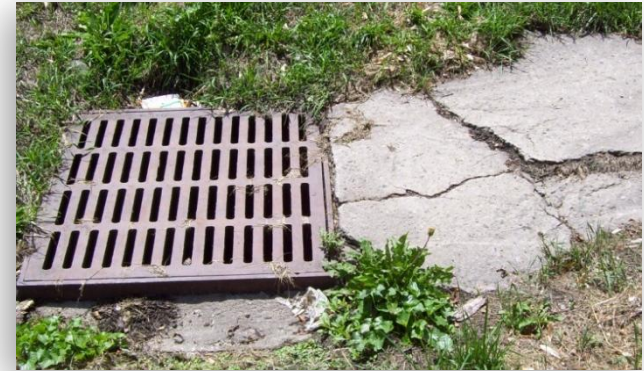
Above: Top view of the outflow grate
