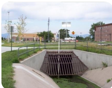
Left: a picture of the grate and water level under normal conditions, notice the algae that could potentially build on grate.
