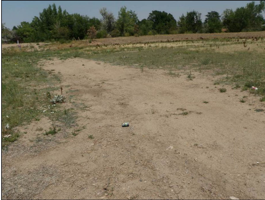
Photograph 23. View facing north at an unstabilized portion of the Central Facility's stormwater retention pond.
