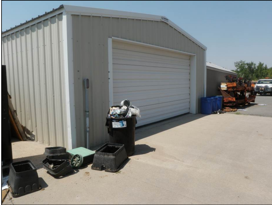
Photograph 21. View facing northwest at a storage area to the east of the Parks and Recreation Storage building at the Central Facility. Note the lack of good housekeeping BMPs implemented to manage the disorganized collection of equipment and the overflowing trash container.
