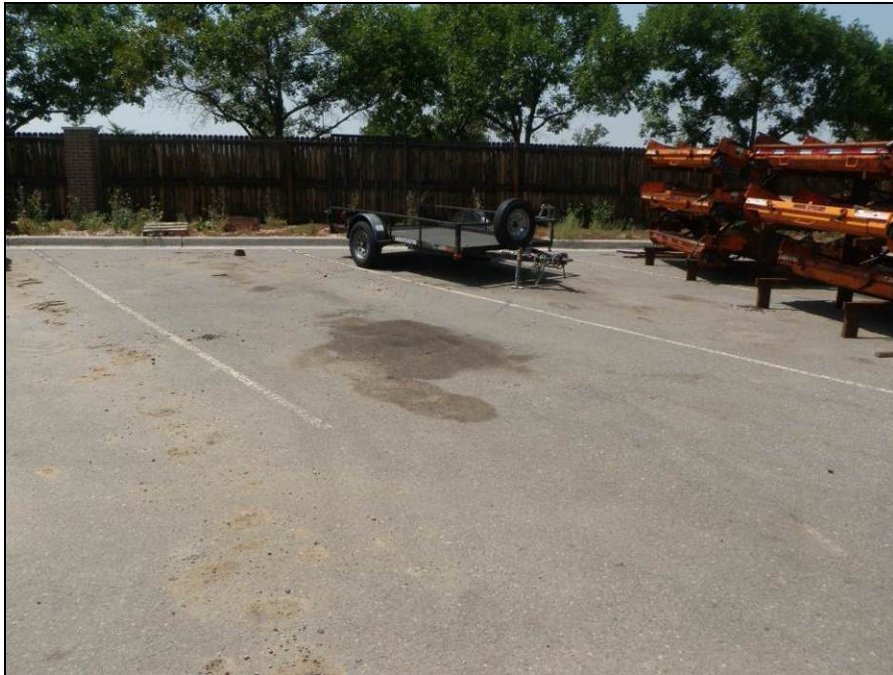
Photograph 18. View facing northwest at outdoor storage area for vehicles in need of repair. Note the petroleum product staining on the impervious surface and lack of spill response BMP implementation.
