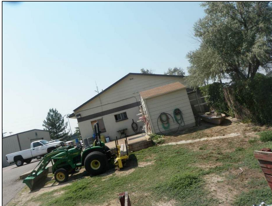
Photograph 14. View facing west at the maintenance building at the Aurora Hills Gold Course. Note that washwaters from the concrete pad in the center of the picture drain to the right (north) of the picture.
