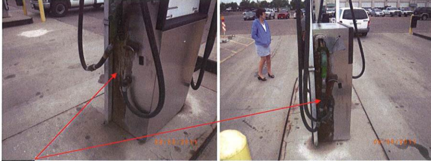
Zone 4 Fueling station pumps observed with excessive spill residues Photo #68, 69
