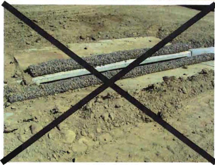
Unprotected inlets can easily be impacted with sediment.
