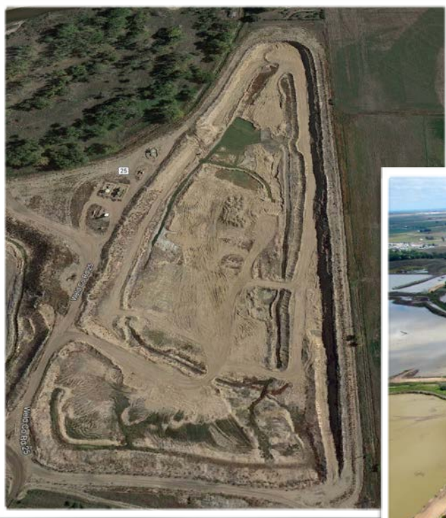
Everist Reservoir (Before)
