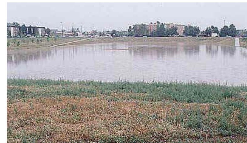
Iliff Stormwater Detention Basin on Goldsmith Gulch
